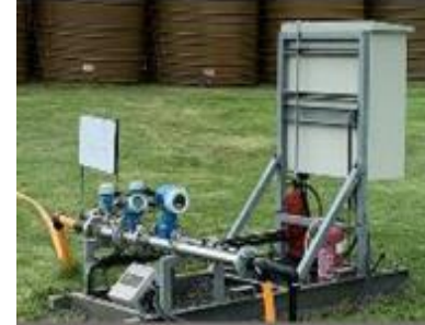
Well head and flow skid
